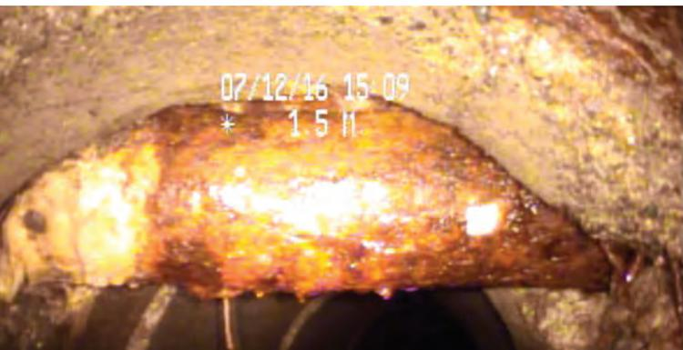
CCTV inspection showed several areas of concern in the sewers, including sections where water lines passed right through the sewer.
